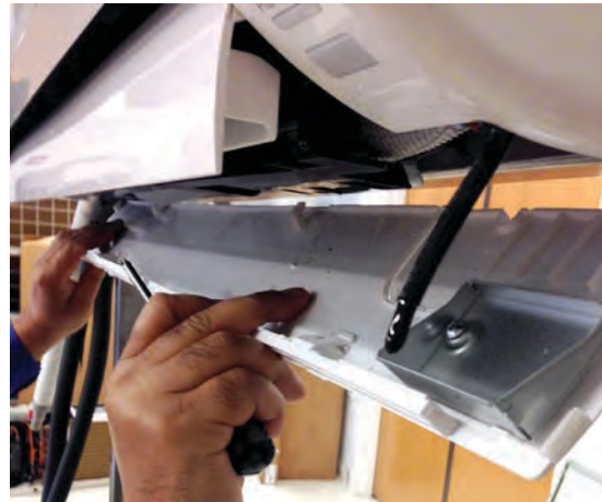
Figure 62: Remove (and Reattachment) Bottom Panel
