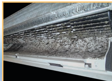
Mold thrives on mini-split blower wheels
